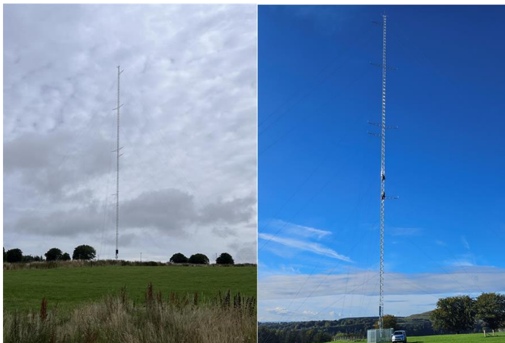
PHOTOGRAPHS OF AN EXISTING MAST LOCATED AT MYNYDD CARN Y CEFN (ABOVE EBBW VALE AND BLAINA)
